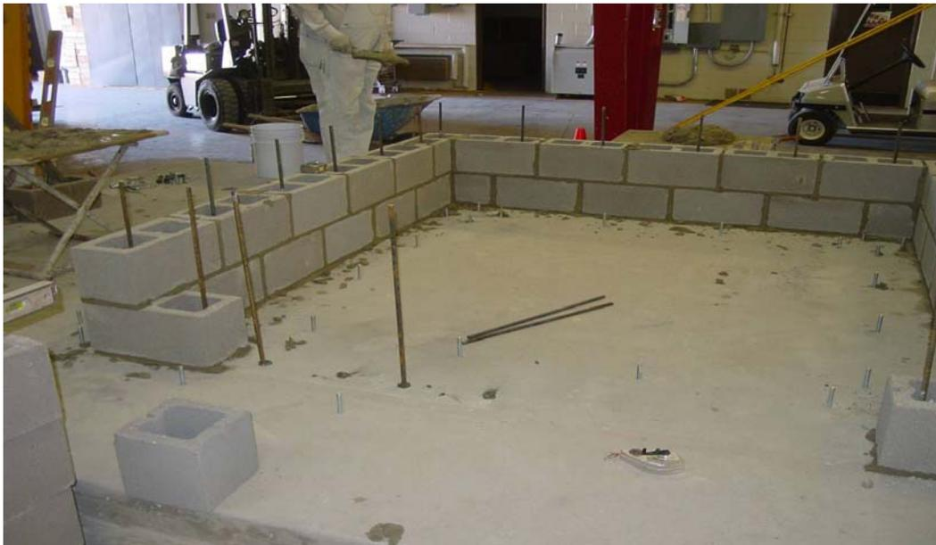
Fig. 7 - Reinforcement within shelter walls
