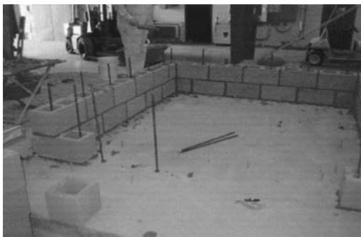
**Fig. 6.** Shelter walls dowels
